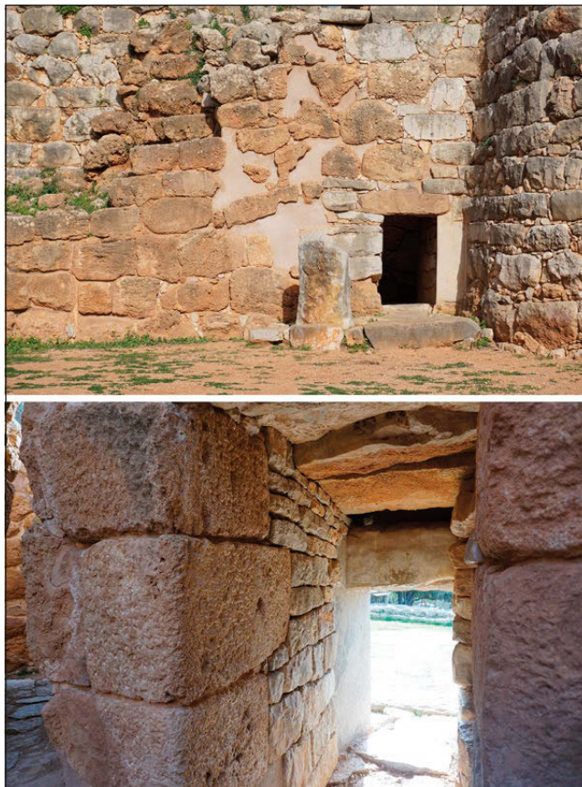
Fig. 6 – Some examples of the recent restoration works carried out on the masonry at the main entrance of the nuraghe.
