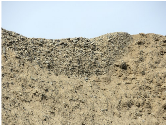
Fig. 9 – The outside of the southern wall of Ciudadela Rivero: the original structure in tapia at the centre and all around it an adobe coating.
